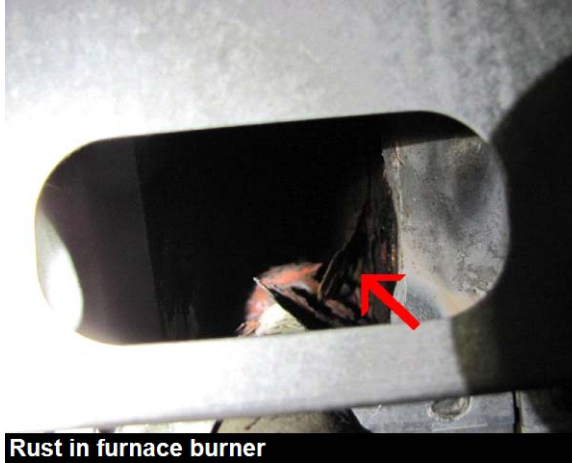
Rust in furnace burner
